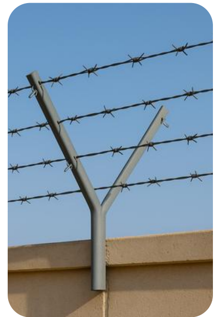
*image of Barbed Wire on Boundary Wall
