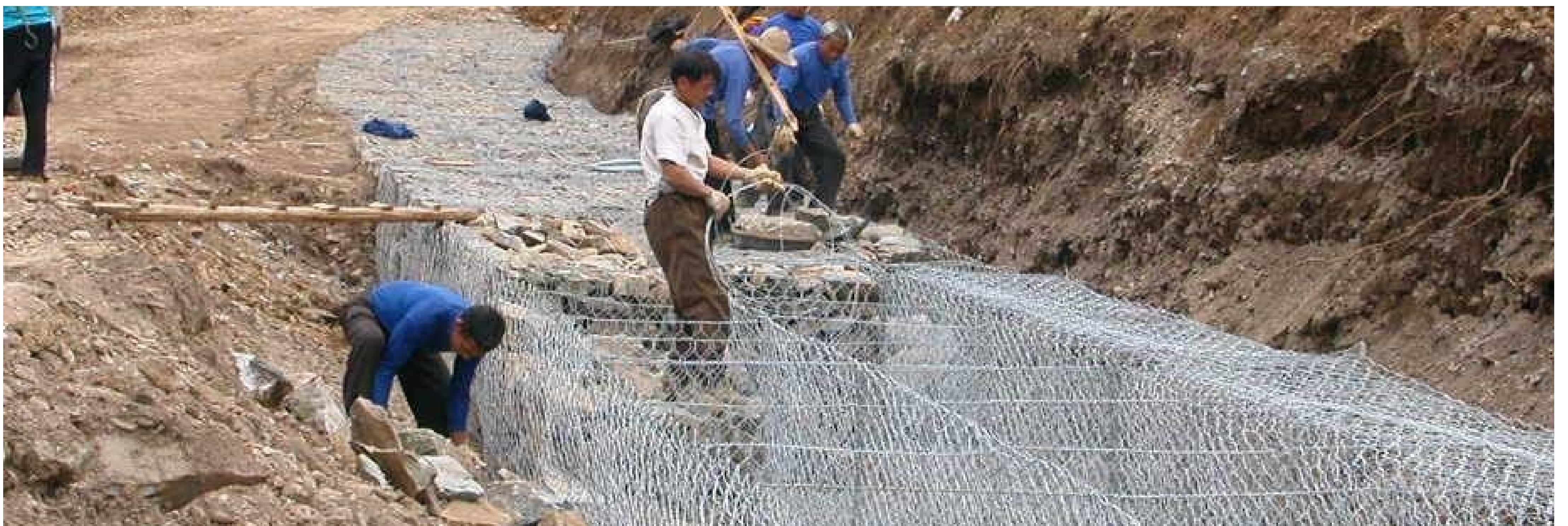
Gabion Protection wall at Road Project, Bhutan
