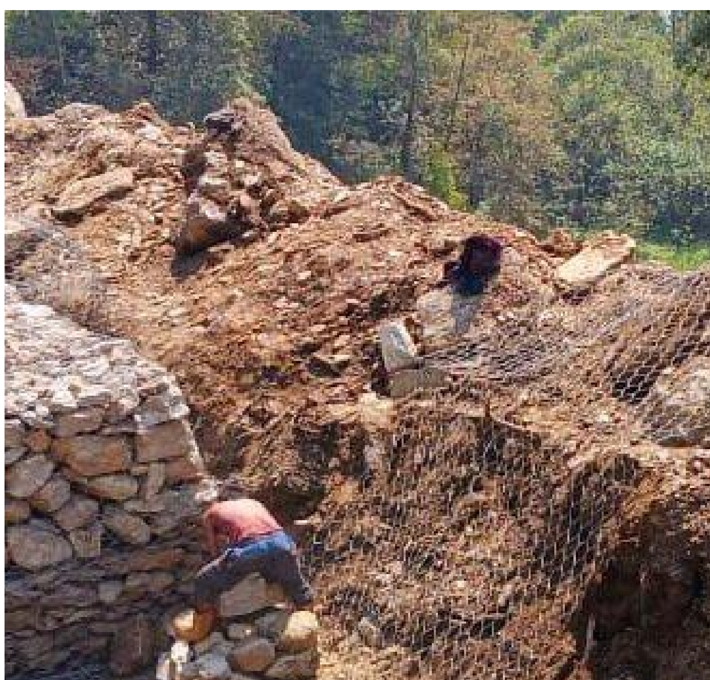
Gabion Wall for NHIDCL Road Project in Sikkim
