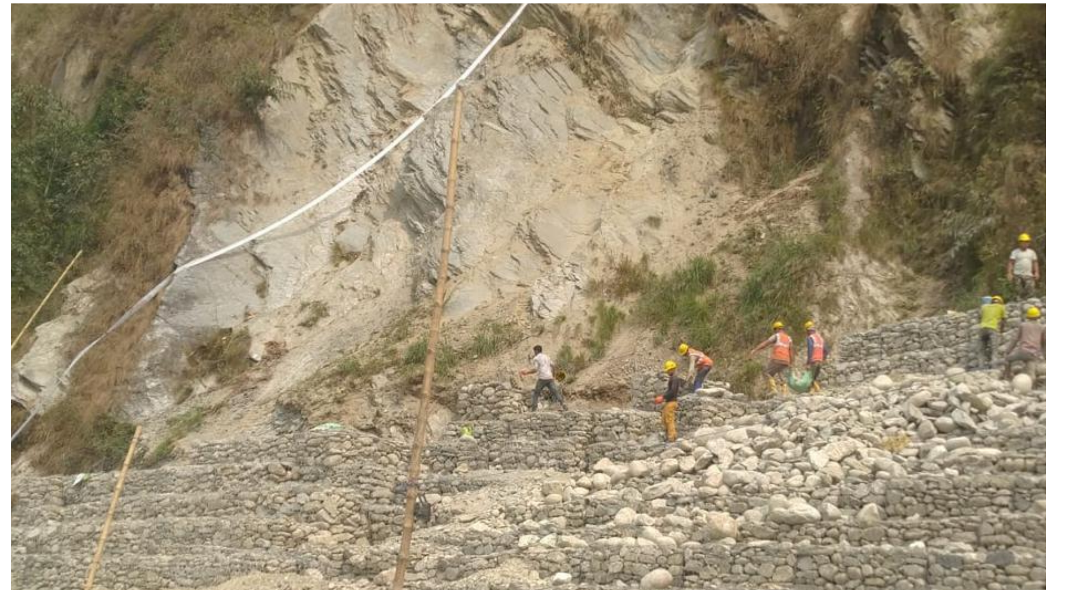
Retaining wall using PVC Gabions for Pharma Unit, Sikkim
