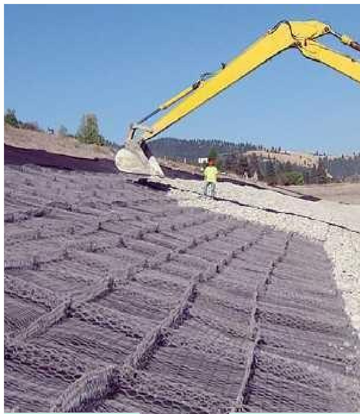
SOIL EROSION CONTROL
