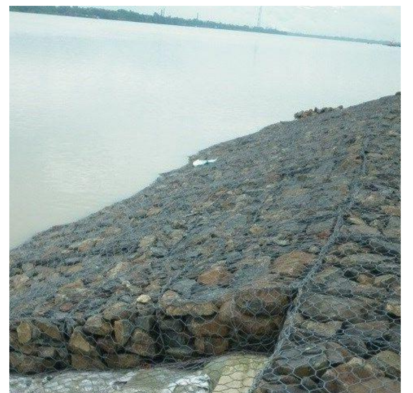
River bank protection using Tirupati Fence® Gabions, Gandak River, Uttar Pradesh
